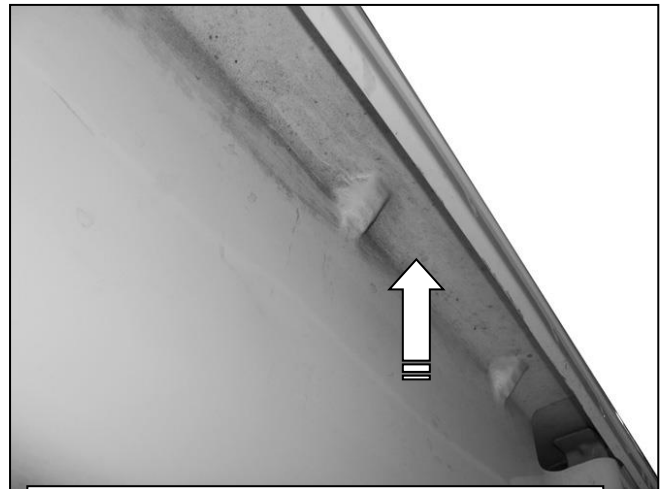
(Fig 10) Before drilling any holes through the top of the bed, check the bottom of the top edge of the bed for hardware clearance.
