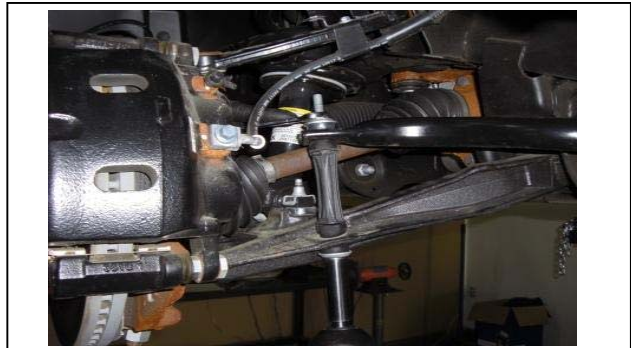
6. Disconnect and remove both sway bar end links.
