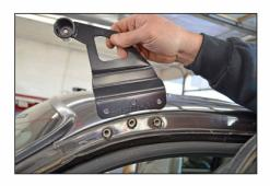
**STEP 8** - Install driver side bracket with the point facing forward.
