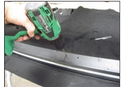
Picture #24: Drill the two scribed holes for the extension bracket.
