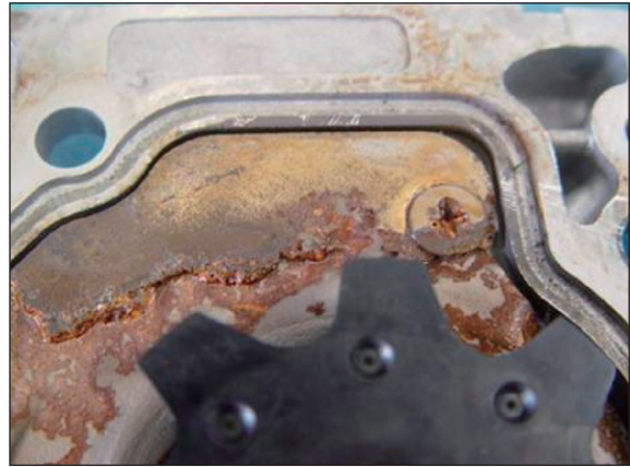
Bottom plate corrosion
