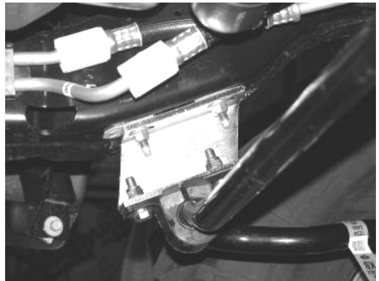
View of inner passenger side frame rail
