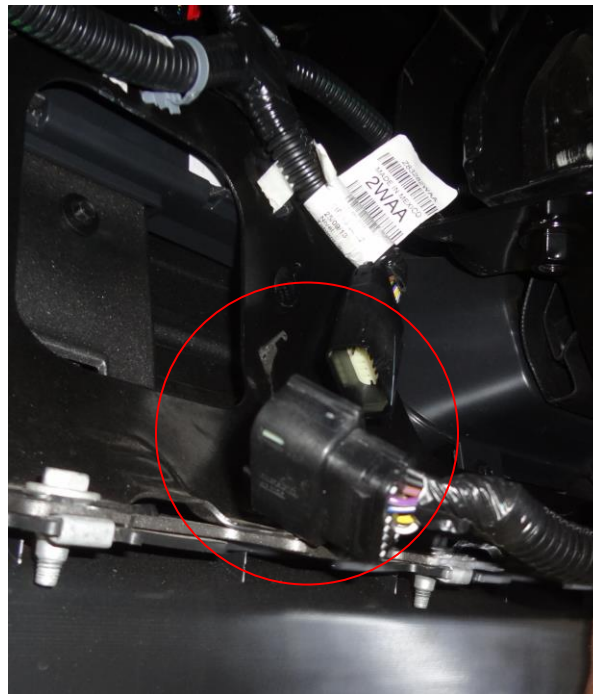
Figure 3(electrical harness disconnected)
