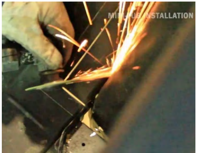
Figure 19 – Cutting the Inside Floor Pan
