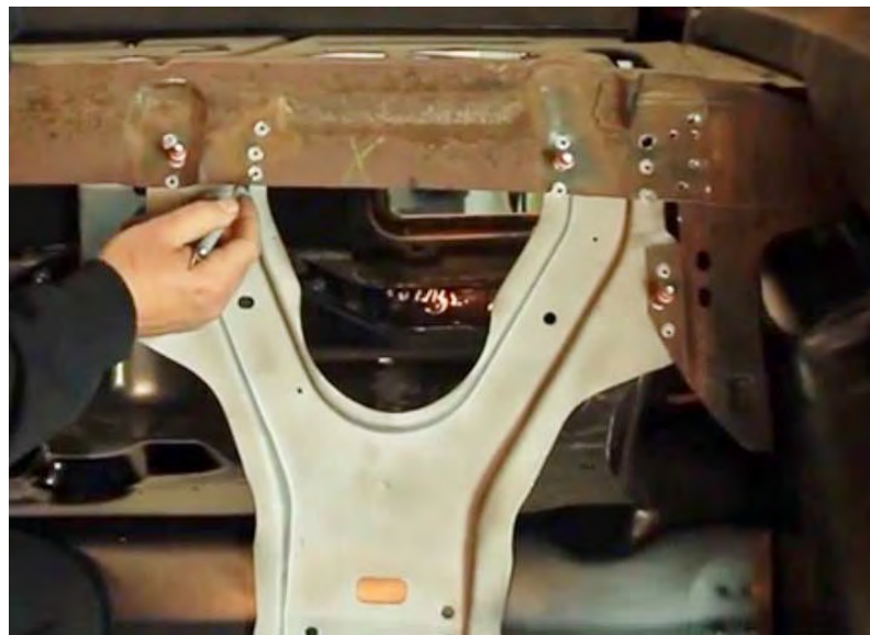
Figure 9 – Drill Out Spot Welds
