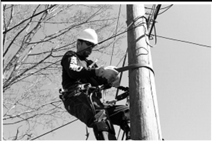
Figure 31 - Reconnect Strap or Lanyard
