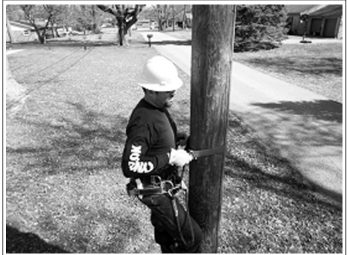
Figure 26 - Climbing Up, Pull Forward
