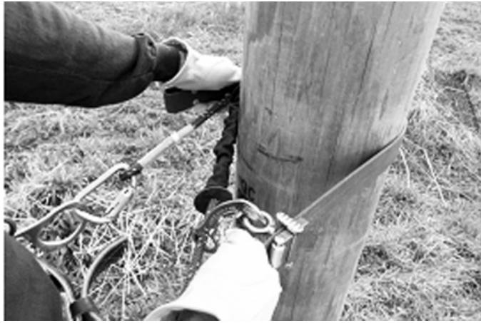
Figure 18 - Two-Handed Adjustment
