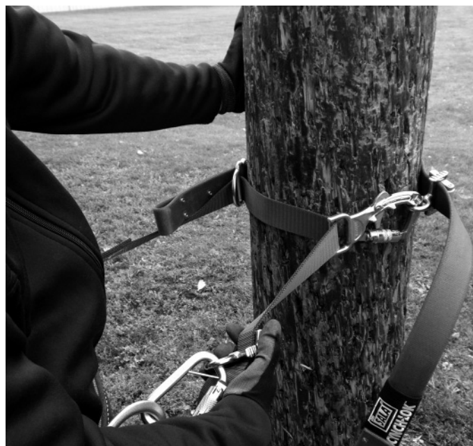
Figure 23 - Adjust Forward into Pole, Web Version
