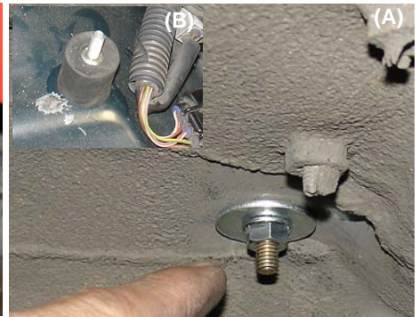
The flange nut and fender washer is fastened to the vibra-mount stud, view from inside wheel well (A). Vibra-mount is now installed, view from engine compartment (B).
