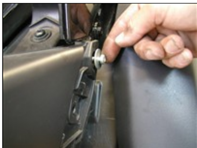
Picture #25: LOWER GRILLE INSTALL
