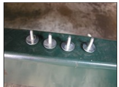
Picture #30: LOWER GRILLE INSTALL
