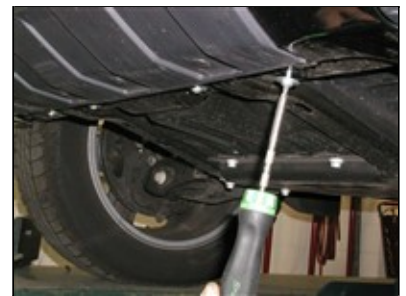
Picture #42: LOWER GRILLE INSTALL
