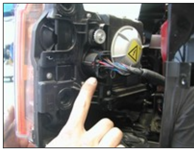
Picture #17: LOWER GRILLE INSTALL
