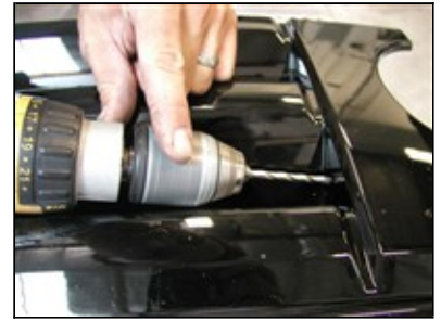
Picture #6: UPPER GRILLE INSTALL.
