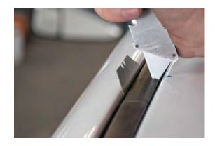
With the molding cut out, place the mounting bracket 'feet' into the opening and mark your holes with a sharpie for drilling.
