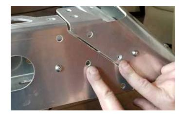
Next, attach reinforcement spacers as shown on all 6 hole locations with provided bolts & nuts. There are three mounting hole locations on each side.
