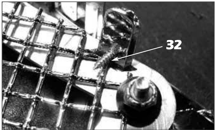
32. Install the supplied #6 x 1/2" countersunk phillips screws through the factory mounting tabs, making sure the screw fits over the mesh wires.
